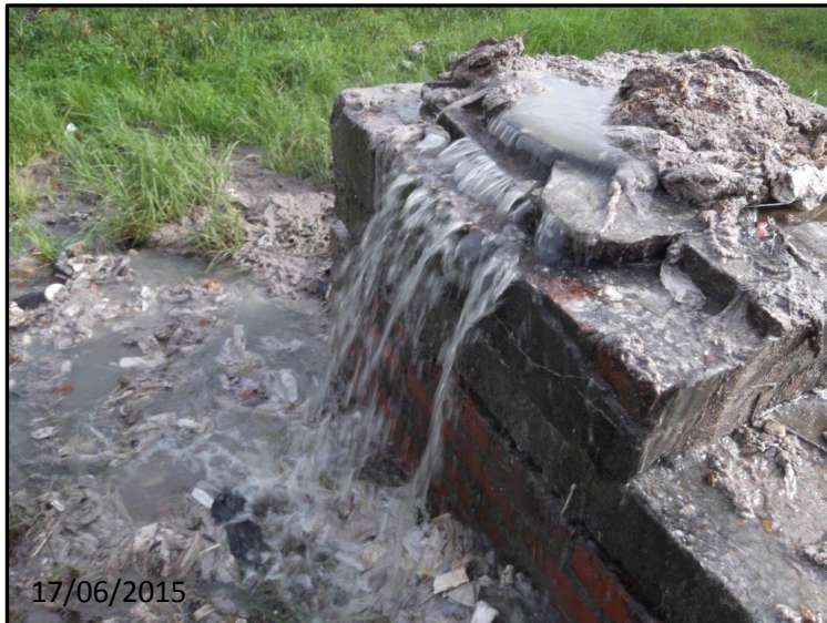
Figure 4: Very recent sewage leak that flowed into the Elsie's River in Da Gama Park.
